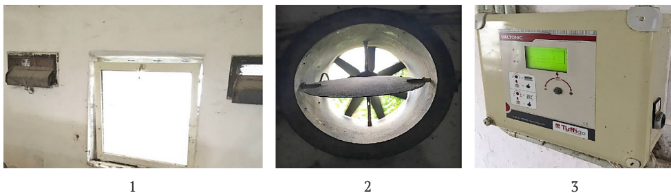
Figure 2. Structural elements of transverse ventilation in the premises for boars of different breeds from the control group
